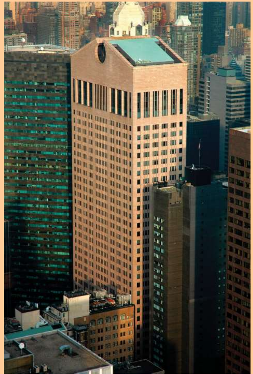
PHILIP JOHNSON and JOHN BURGEE AT&T (now Sony) Building, New York, 1978-1984.
