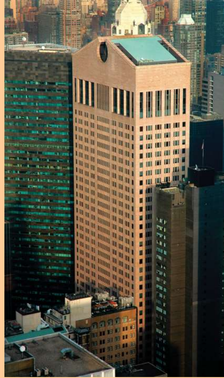
PHILIP JOHNSON and JOHN BURGEE AT&T (now Sony) Building, New York, 1978–1984.
